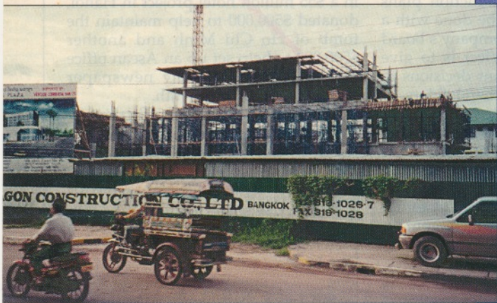
Faces of Vientiane: new construction at the city centre (above); the Monument of the Dead (right), honouring the military heroes of Laos.
